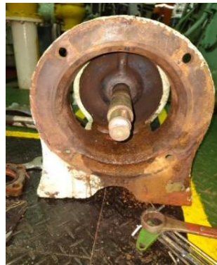
Gambar 4. Overhaule Pompa
