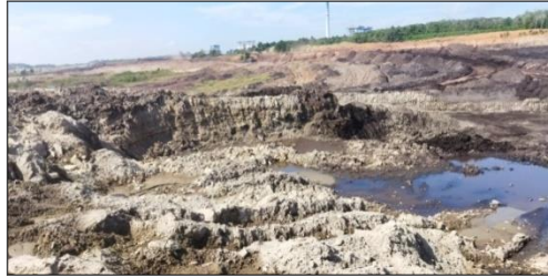
Figure 4.9 Landslides in the Excavation Area
